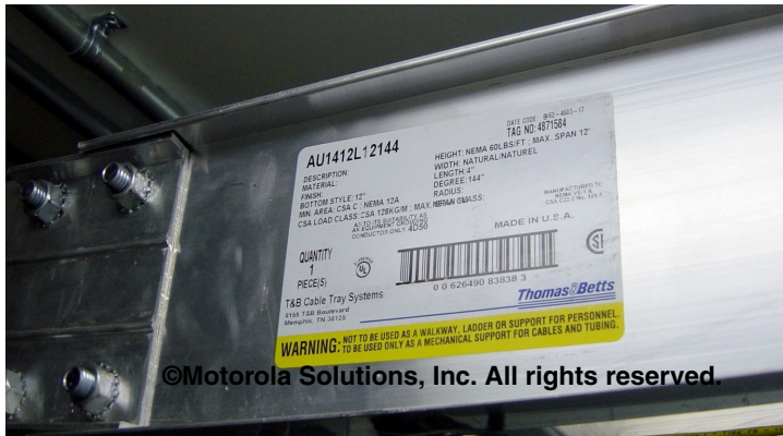
Figure 5-96 Cable Tray Listed as Equipment Grounding Conductor
