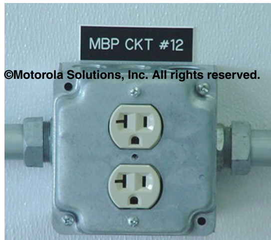
Figure 6-6 Receptacle Circuit Identification
