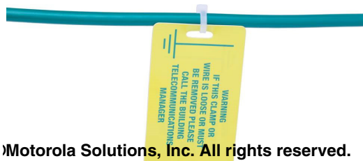
Figure 5-24 Secondary Bonding Bar Grounding Electrode Conductor Identification
