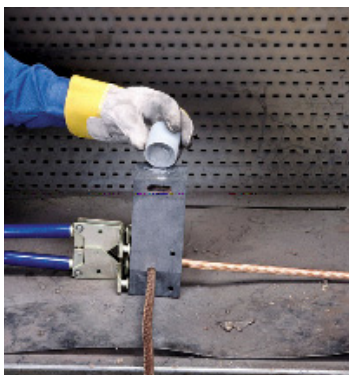
STEP 4: Sprinkle starting material over the weld metal and close lid.
