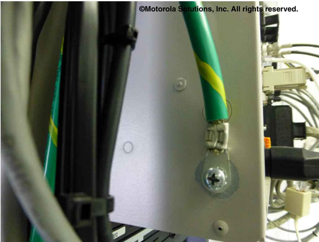
Figure 5-89 Example of Equipment Bonding - Channel Bank
