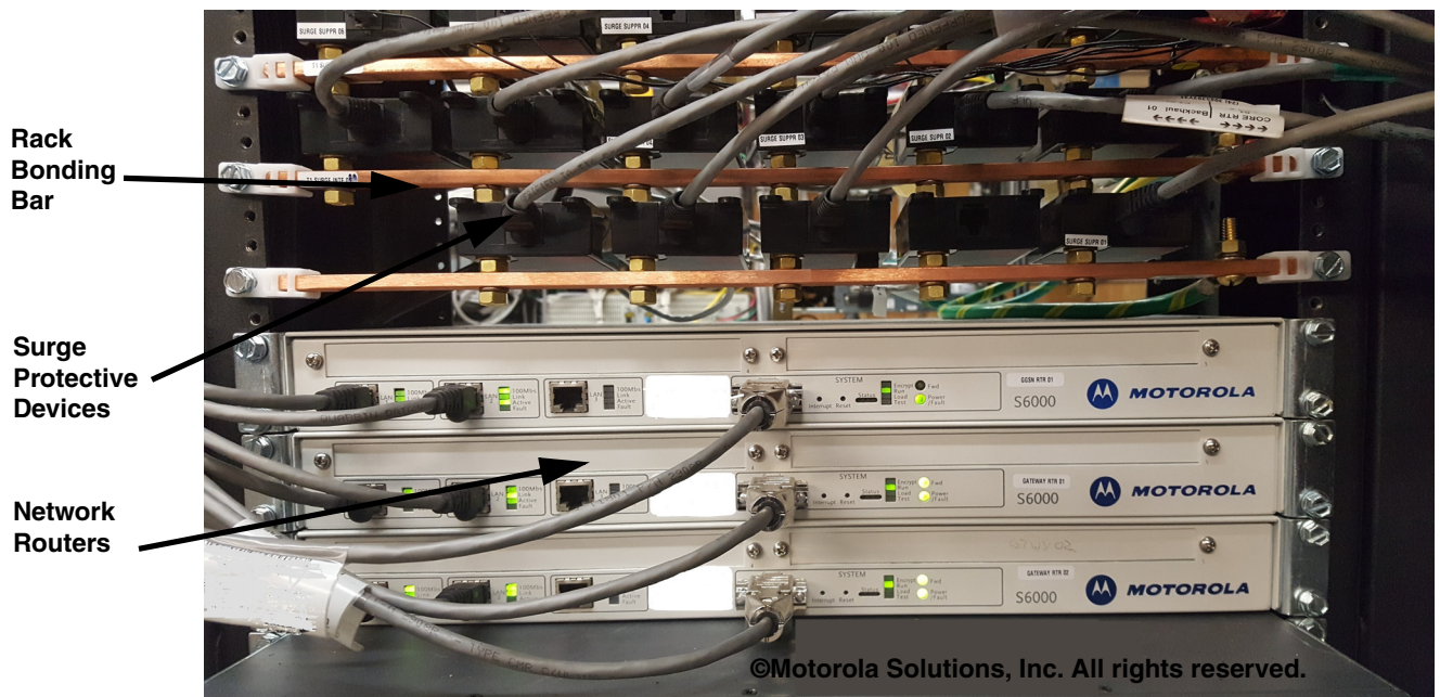
Figure 7-16 Secondary Surge Protective Devices Installed Near Protected Equipment
