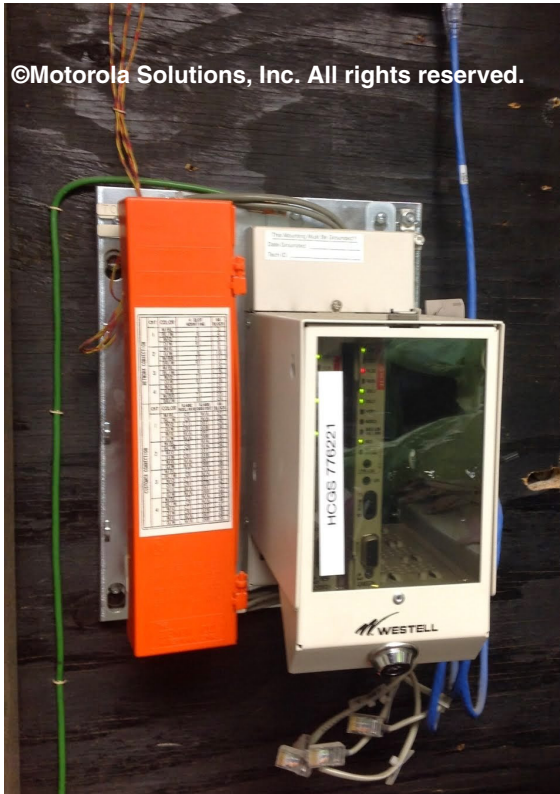
Figure 7-15 Example of Service Provider Demarcation (Network Interface Device)
