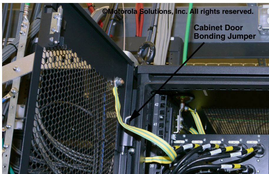
Figure 5-47 Example of Cabinet Door Bonding Jumper
