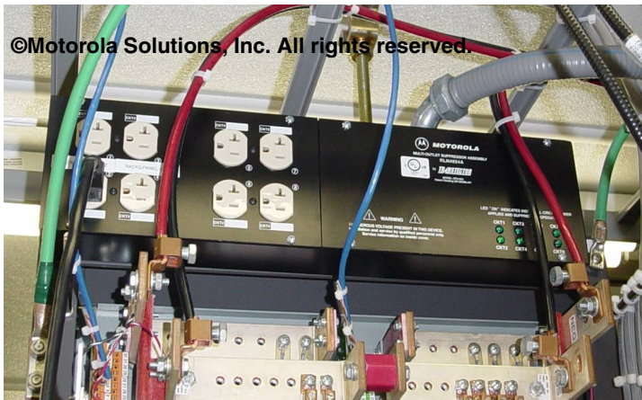
Figure 9-28 Example of Rack Mounted Receptacle Assembly
