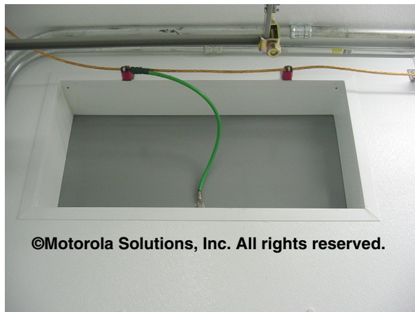
Figure 5-108 Example of Bonding Unused Entry Port to Internal Perimeter Bonding Bus
