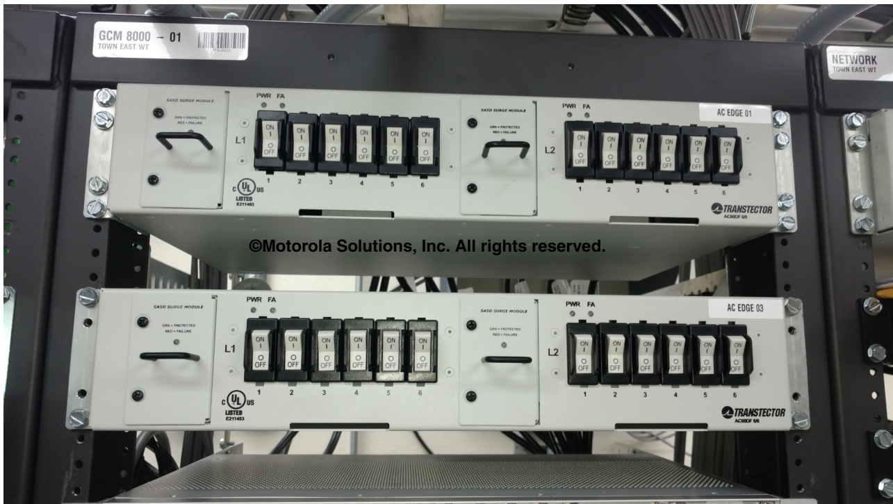
Figure 7-10 Example of Rack Mounted Power Distribution Unit with Type 3 SPD
