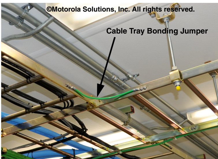
Figure 5-46 Examples of Bonding Cable Tray Sections
