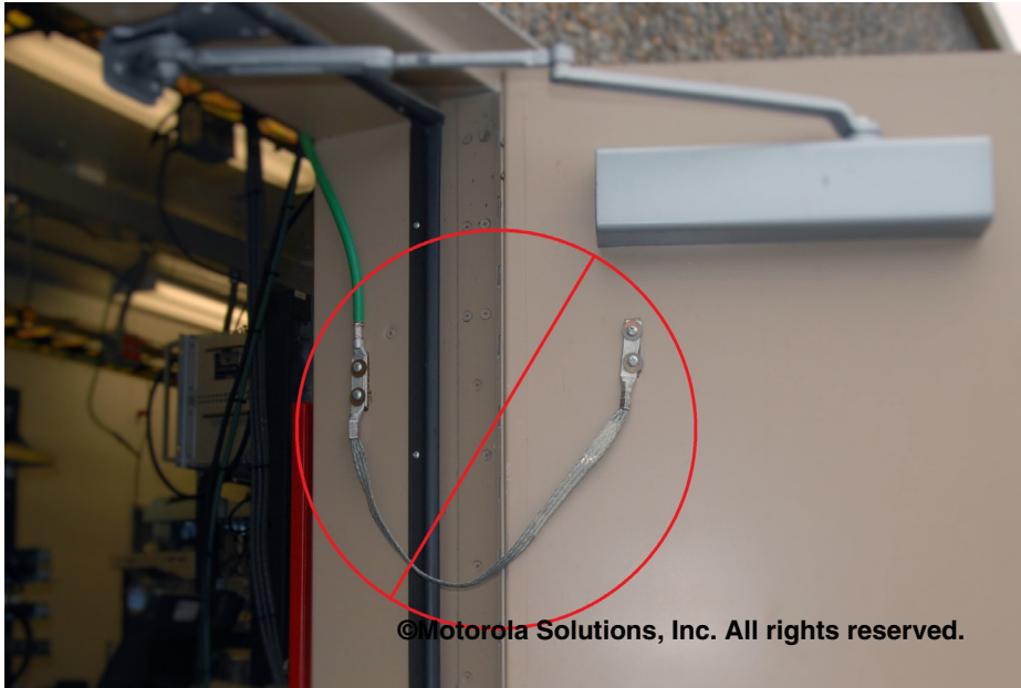
Figure 5-45 Improper Use of Flat Braided Bonding Conductor
