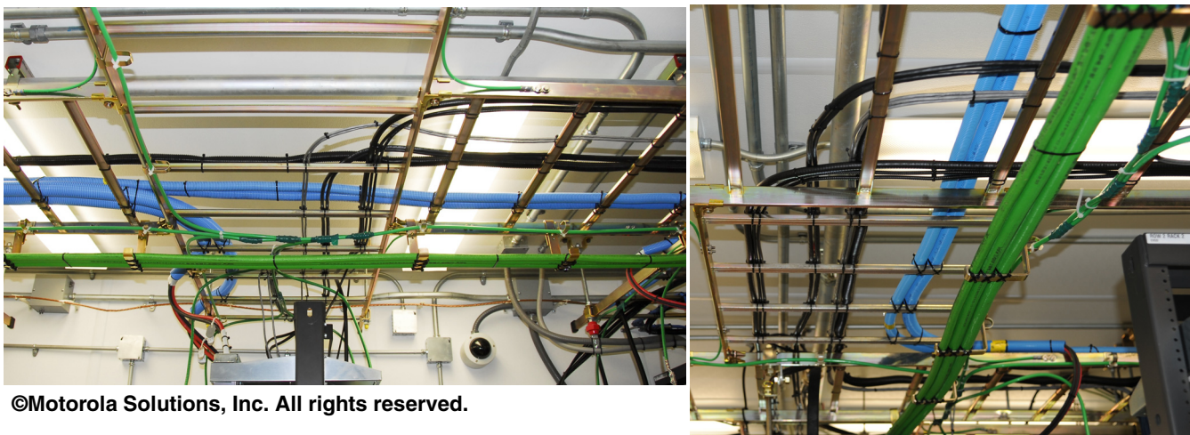
Figure 9-25 Proper Securing of Cables in Cable Tray
