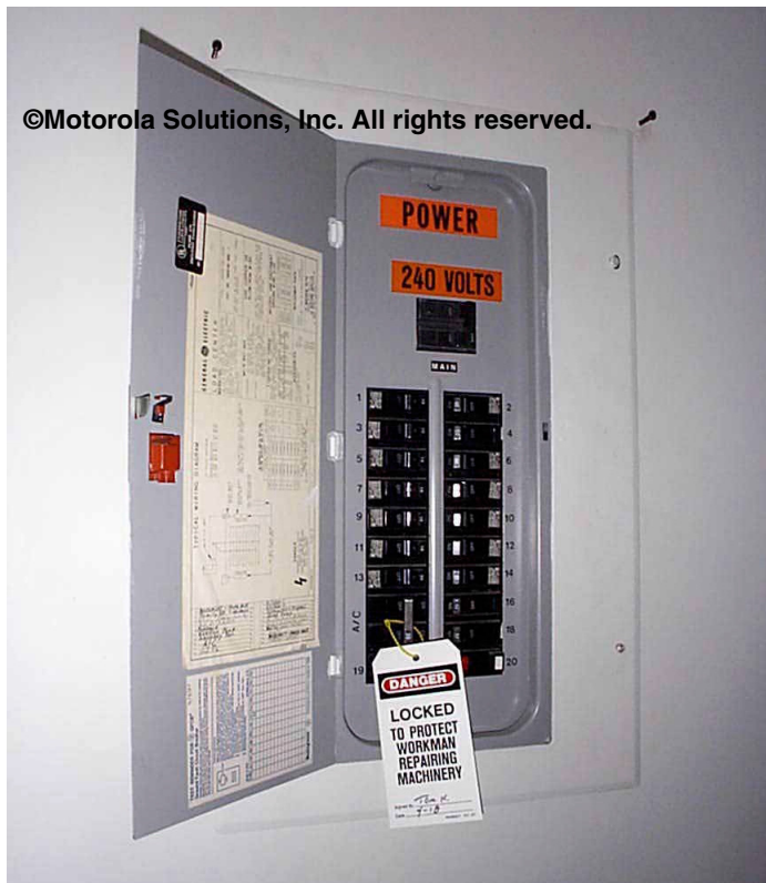
Figure 6-1 Proper Tagout of Circuit
