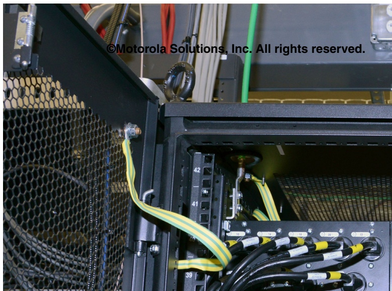
Figure 5-93 Example of Removable Cabinet Door Bonding
