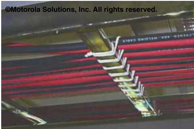
Figure 9-48 Example of Cable Lacing for a Utility
