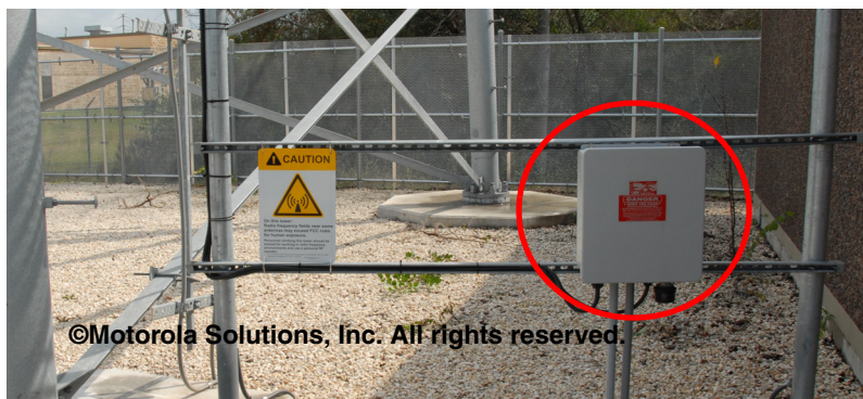
Figure 7-38 Tower Light Controller Installation
