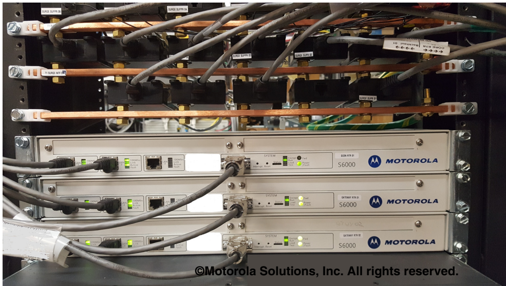
Figure 5-119 Surge Protective Devices Installed at Equipment Rack or Cabinet
