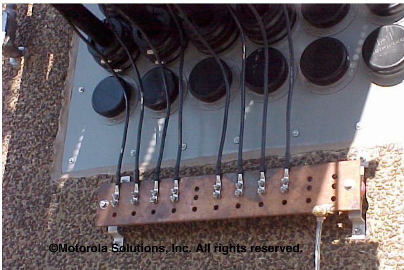
Figure 3-4 Single-Point Grounding at Entry to Building
