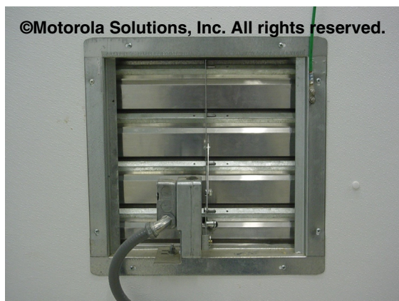
Figure 5-105 Example of Exhaust Louver Bonding
