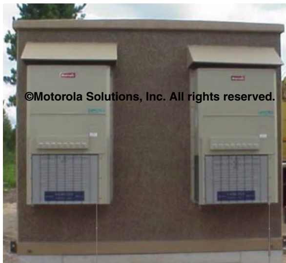
Figure 3-7 Typical Commercial Wall-Mounted Air Conditioning Unit
