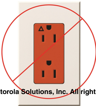
Figure 5-142 Example of Unapproved Isolated Ground Receptacle (Orange Colored)
