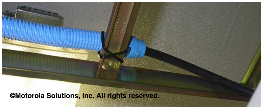
Figure 9-30 DC Power Conductor Routed in ENT
