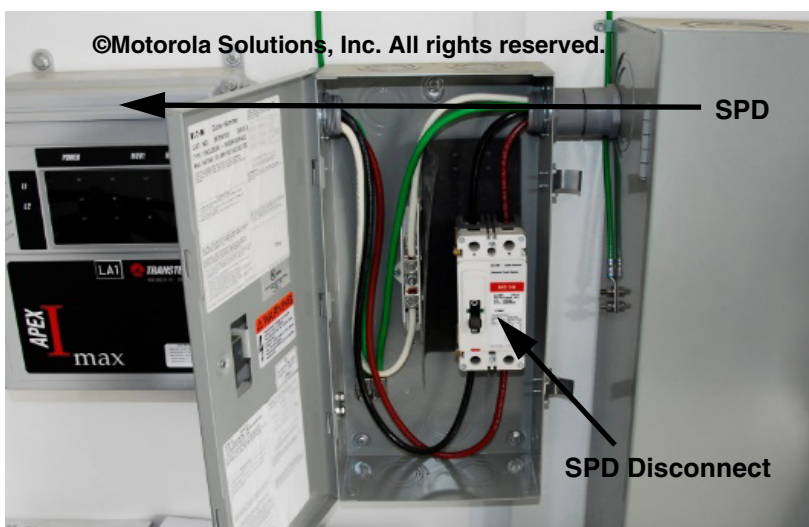
Figure 7-11 Example of SPD Exterior Disconnect
