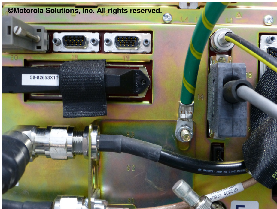
Figure 5-88 Example of Equipment Bonding - Base Station/Repeater
