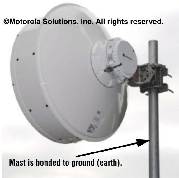
Figure 7-22 Example of Broadband Wireless Radio
