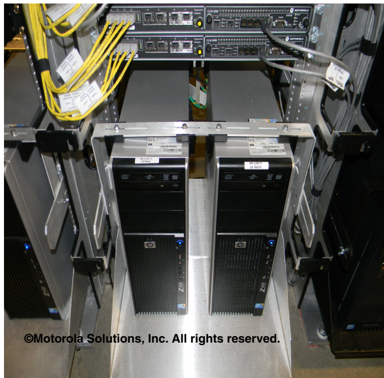
Figure 9-16 Example of Securing Equipment
