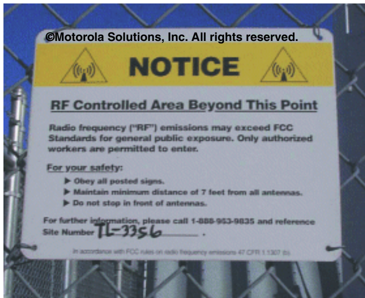
Figure 3-19 Typical RF Warning Sign
