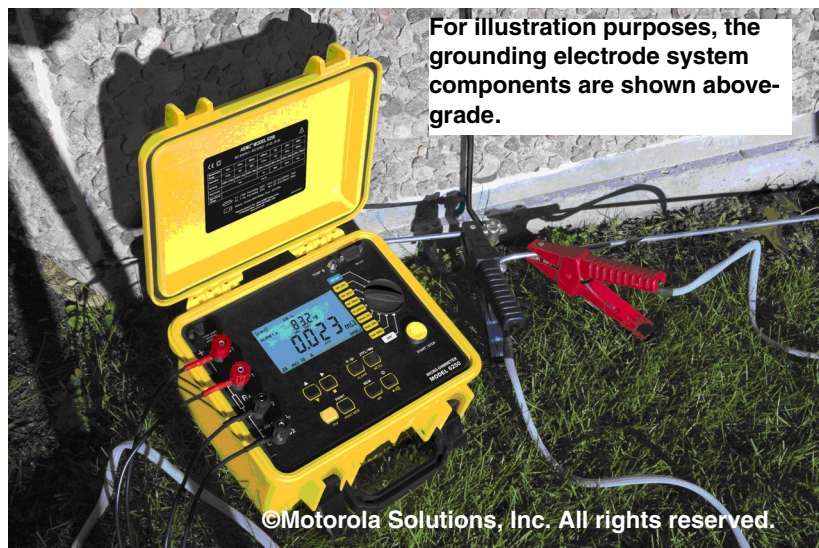
Figure 4-59 Example of Micro-ohmmeter Testing
